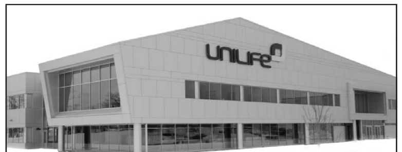
Recently completed: Unilife Medical Solutions New World Headquarters, a Pennsylvania-based medical device company.
